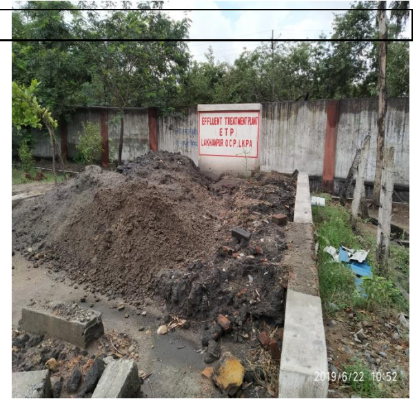
Sludge drying bed
