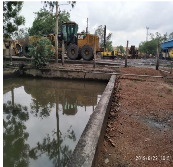
Sedimentation tanks
